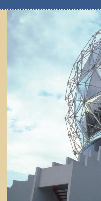
**SCIENCE WORLD** This building was constructed for the Expo '86 World Fair held in Vancouver, British Columbia. The structure is a geodesic dome containing 766 triangles.
