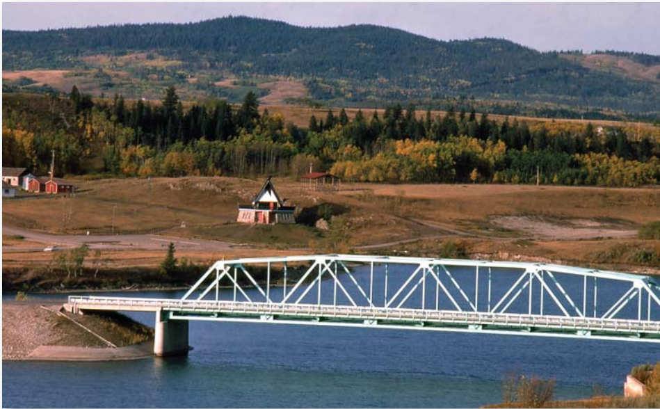
Truss bridge over the Bow River in Morley, Alberta located on Chiniki First Nation territory.
