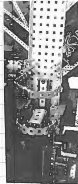
The Replaced Motor
