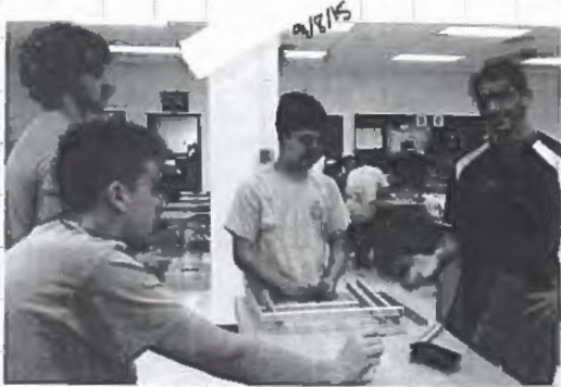
Building the Base's Frame
